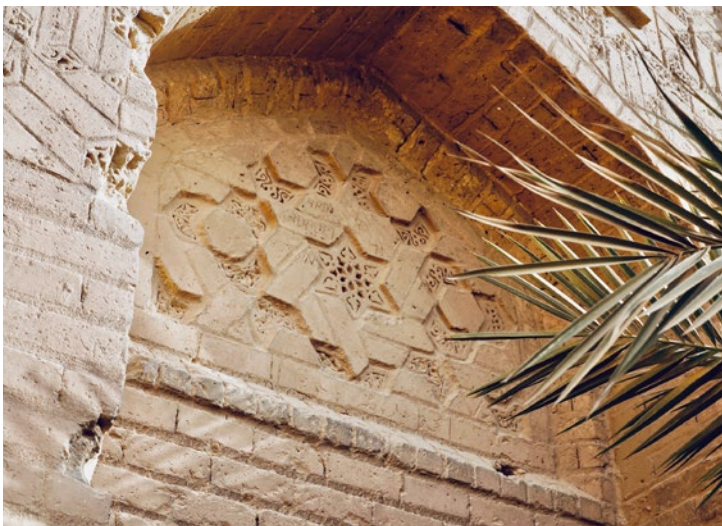
House formerly inhabited by Jewish families. The majority of Jews left Iraq in the period between 1949-1951 due to political and economic insecurity. Baghdad, Iraq | 2022
