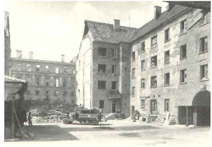
20 The courtyard of the post building before repairs, a guard at left and guard vehicle at center.
