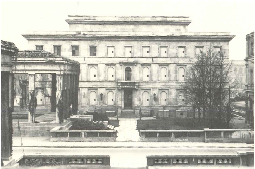
21 Gallery II (the renamed Führerbau) with newly filled windows of storage rooms.
