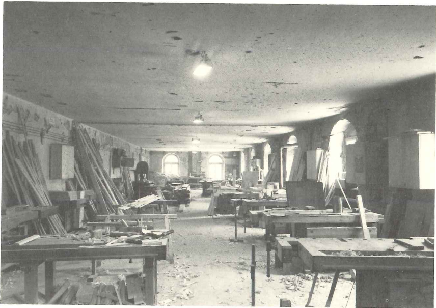
22 Carpenter shop, newly set up in the Power House.
